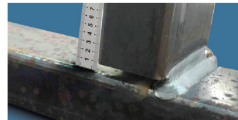
Mild steel / fillet Thickness 2mm, current 110A Unified voltage Clearance 3mm, welding speed 50cm/min
